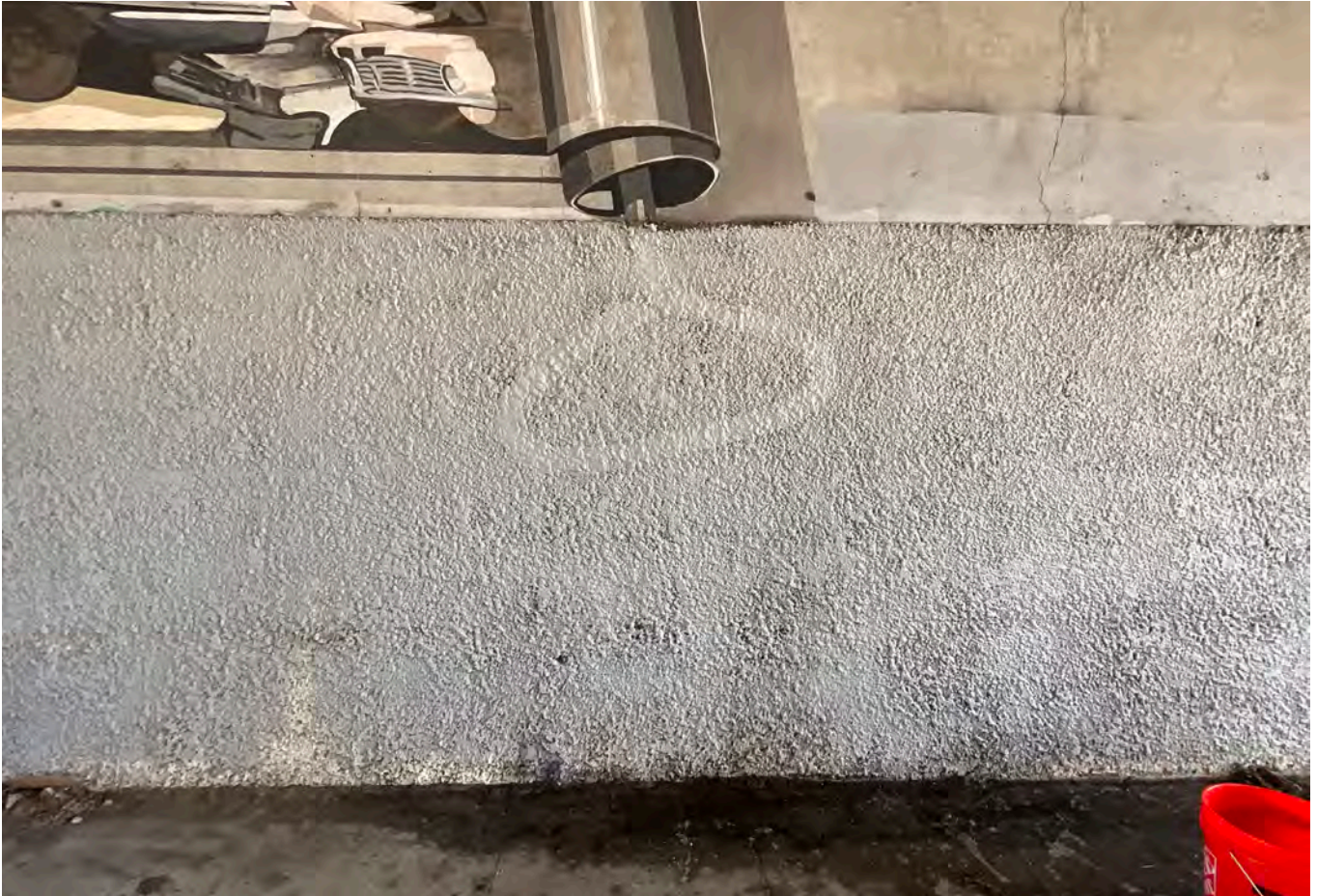
Figure 3. Before treatment, July 2024. The key and it's shadow have been obscured by 7 layers of graffiti and overpaint.
